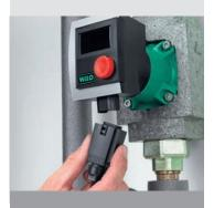
The plug connection can then be connected to the pump with one simple hand motion.
